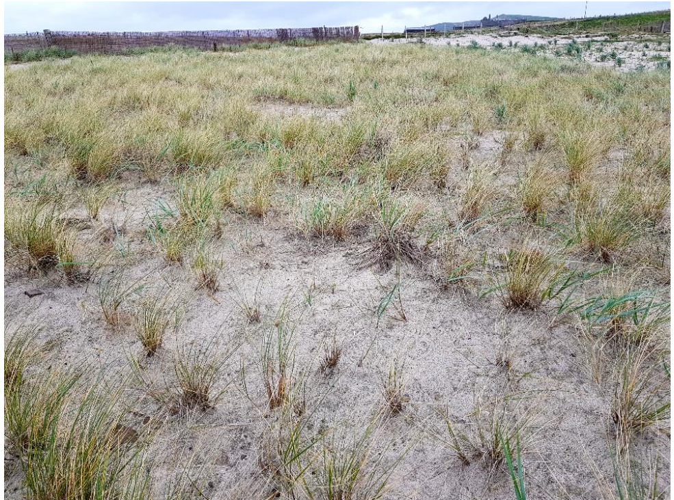
Figure 12b: Dune stabilisation works at Links of Noltland commenced in 2011 has involved the re-planting of Marram and Lyme grasses to try and restore the natural protection of the dune system. (Copyright Historic Environment Scotland.)
