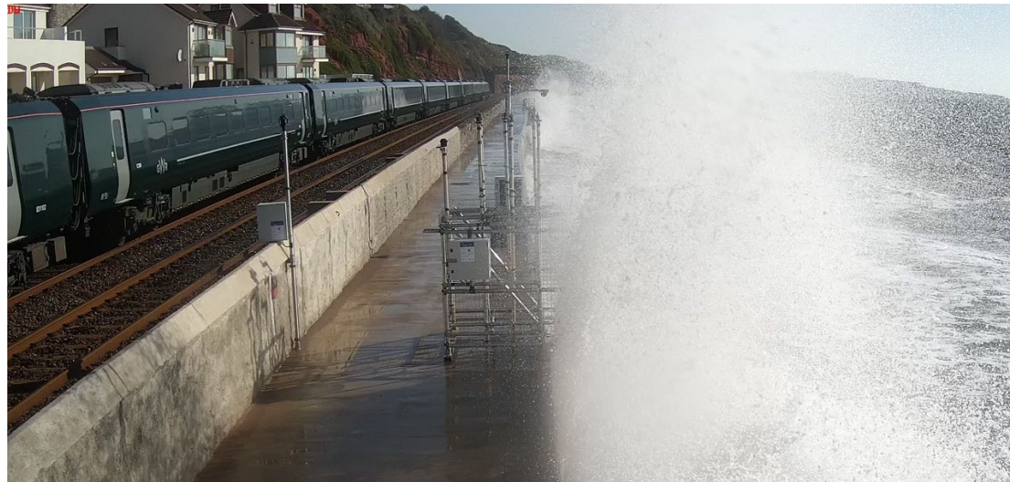
Figure 3: A hard-engineered coastline with railway infrastructure and a new wave overtopping measurement system, “WireWall”. Photo from the University of Plymouth’s Dawlish camera installed as part of the Coastal REsistance: Alerts and Monitoring Technologies (CreamT) project.
